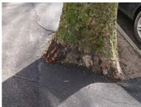
Figure 1 A ring at the tree’s base shows the tarmac level before the many built-up layers were removed.
