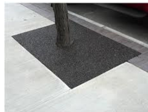
Figure 2 Flexi™-pave is a tarmac alternative that is used around tree roots and is standard practice in many cities.
